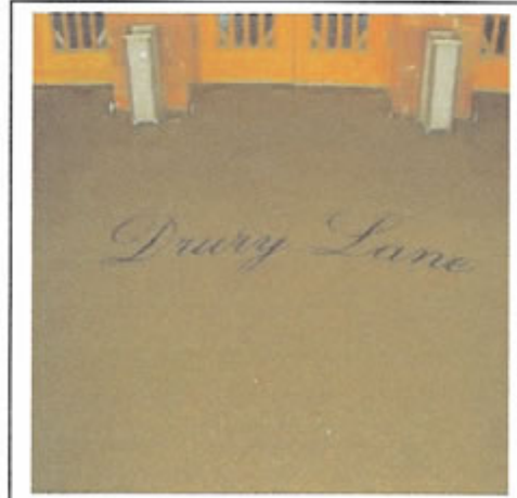
The grit system compliments this theatre entrance way with brass terrazzo strips and black grit.
