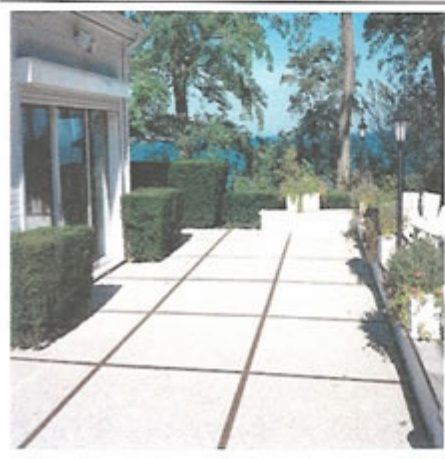
The ROYAL LINE RESIN grit SYSTEM adds the final touch to this lake front property with two colors.
